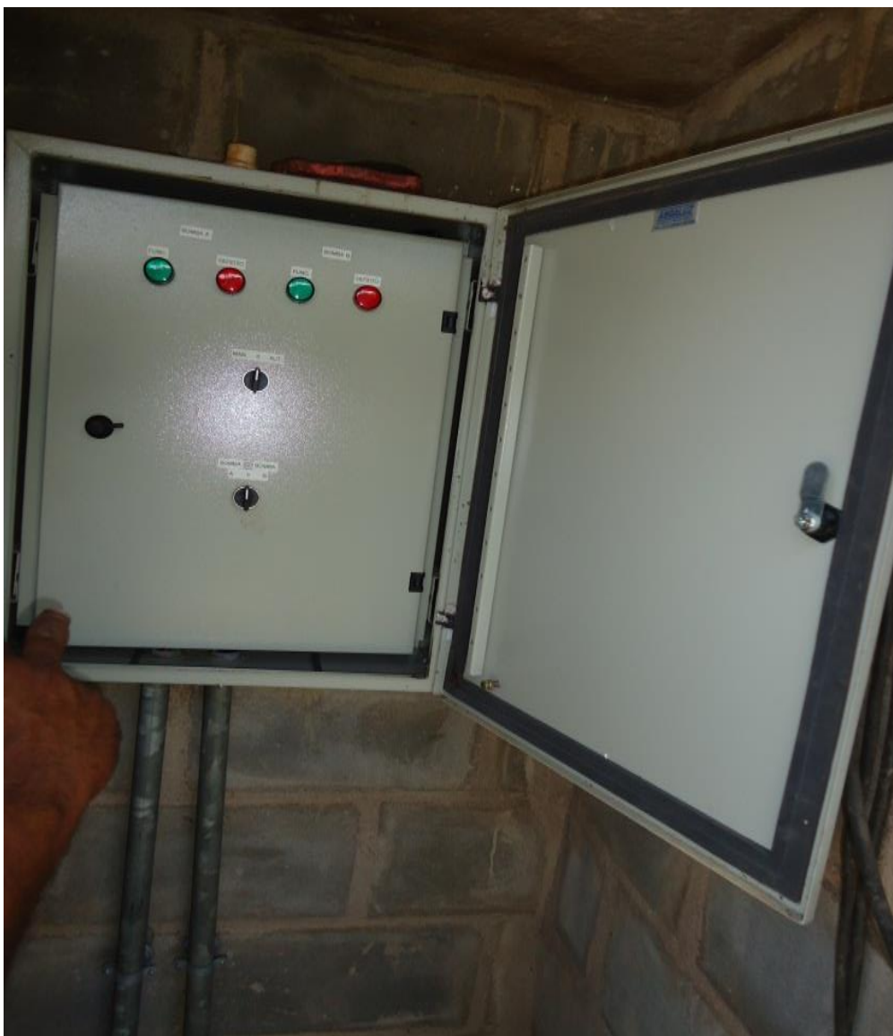
Figura 106 – Painel de Controle.
