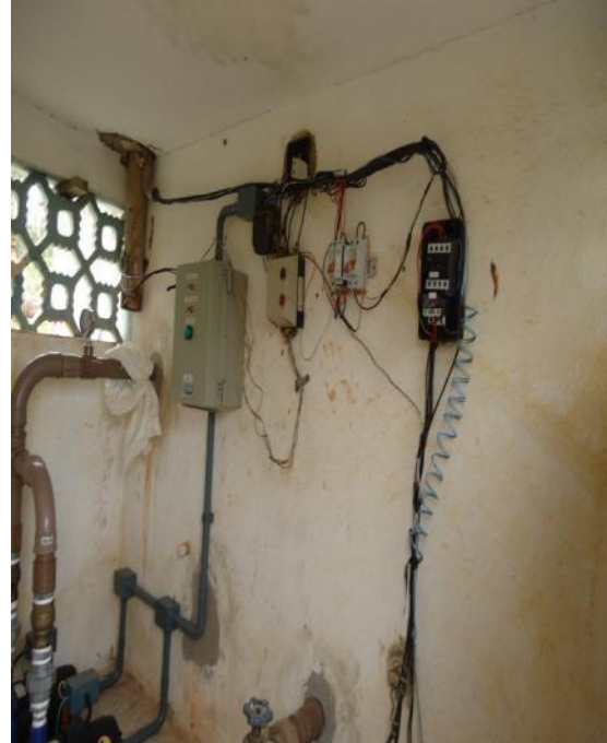
Figura 91 – Painel de Controle EEAT.
