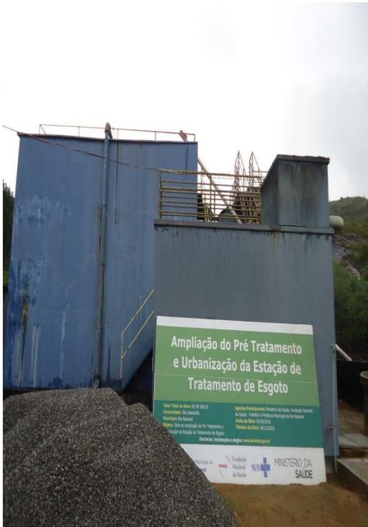
**Figura 187- Reator UASB.**
