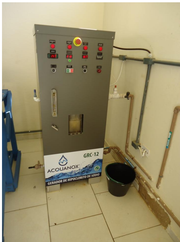
Figura 19 – Painel de Controle.
